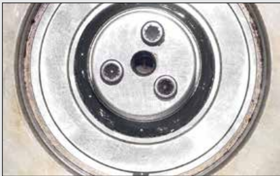
Fig. 66. "Clean" grease slightly purging (leaking) from a bearing during initial start-up is generally acceptable. The grease is wet and evenly purged. If this slight purge is not causing any problems, leave it alone as it is an effective barrier seal.
